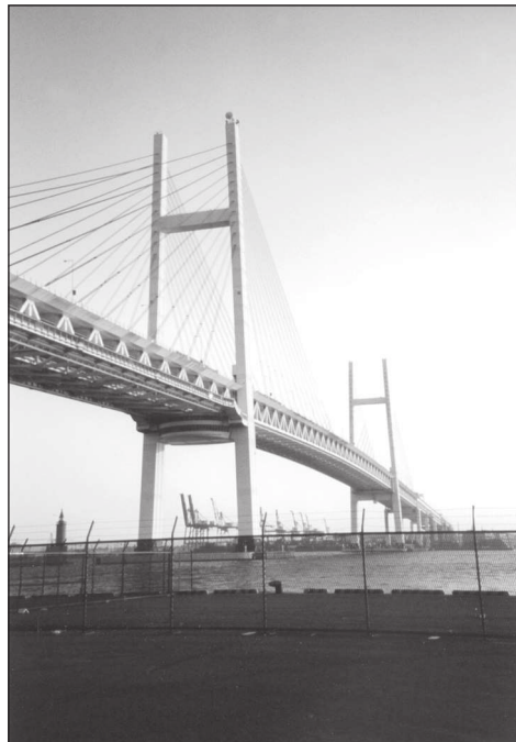
Figuur 1.3. Yokohama Bay Bridge te Yokohama, Japan.
